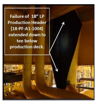
Recently, an 18-in low pressure production header on a producing platform in the Gulf of Mexico failed under normal working pressure. The failure ruptured the header, opening a 10-ft long split and releasing production fluids at a pressure of 250-psi. Three workers were sprayed with production fluid and approximately 25 bbls were released. The event resulted in the evacuation of the platform.
