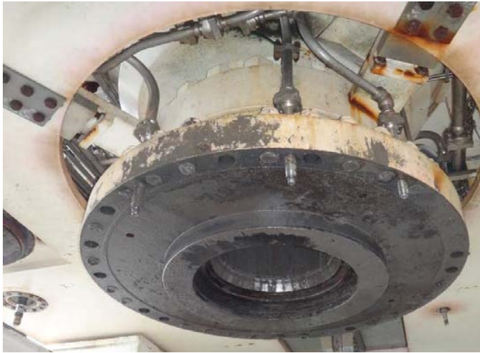
Upper half of failed LMRP Connector
