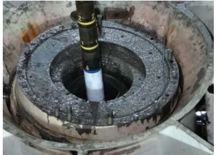
Lower half of failed LMRP Connector
